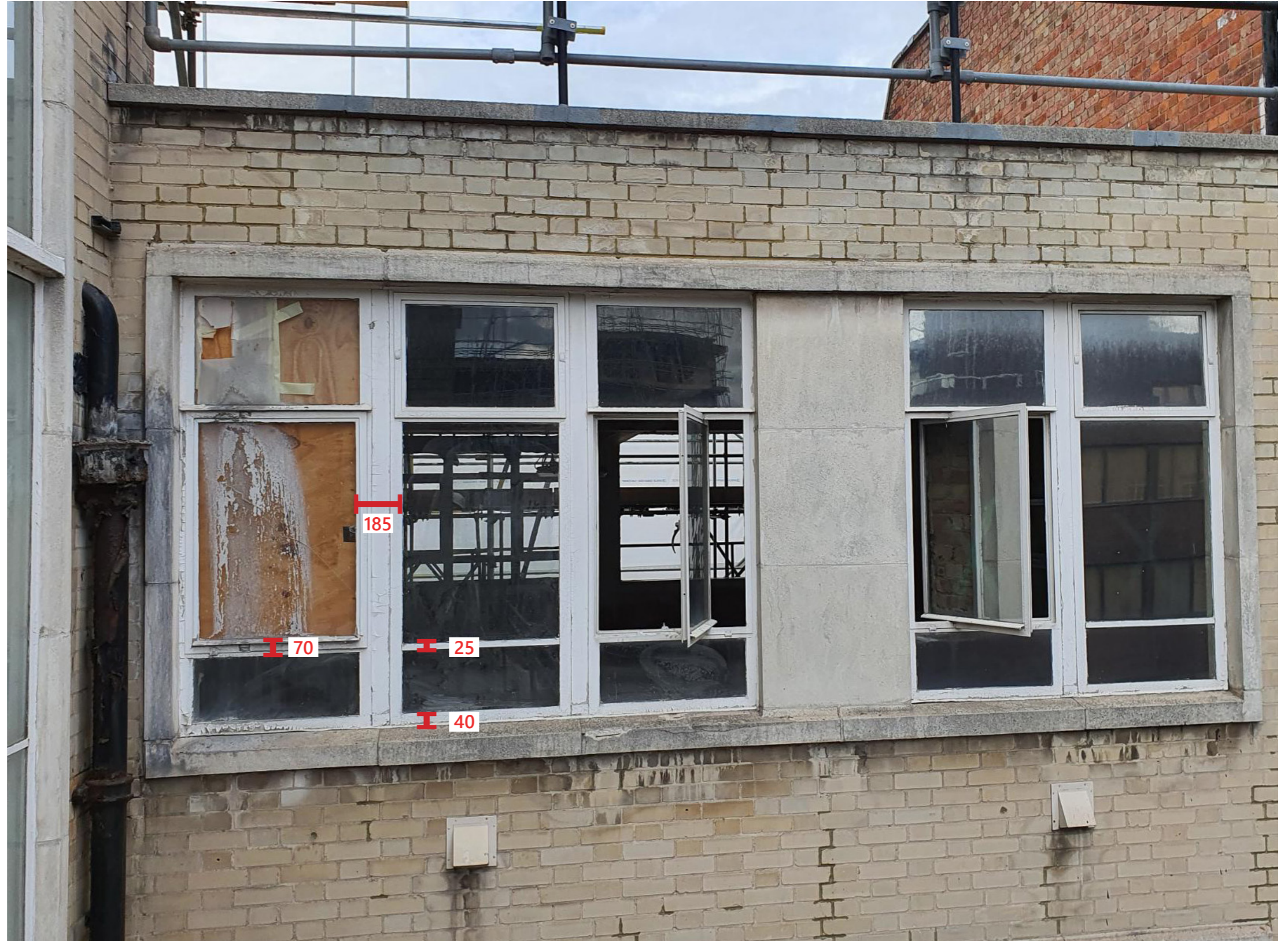
Image of existing single glazed window to be replaced
