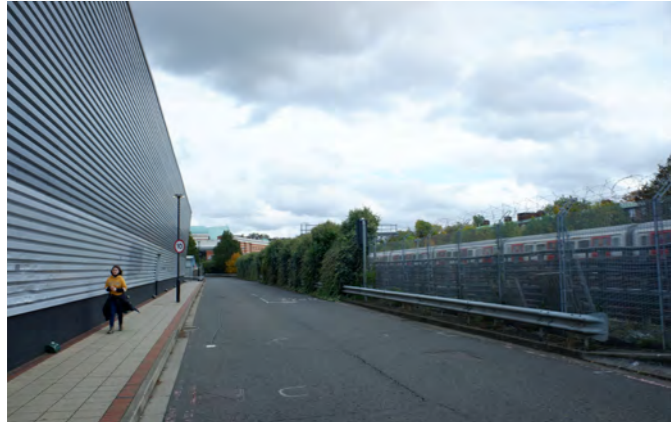
Service road towards West Hampstead
