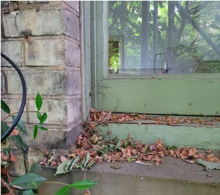
STONE SILLS BENEATH WINDOWS APPEAR TO BE IN GOOD CONDITION AND WILL BE REPAIRED AS NECESSARY AND RETAINED.
