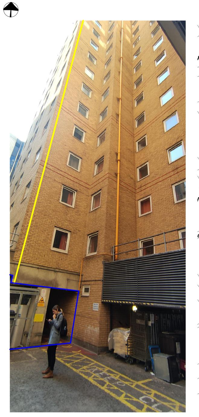
Route of existing and location of new flue pipe to be installed (yellow line)
