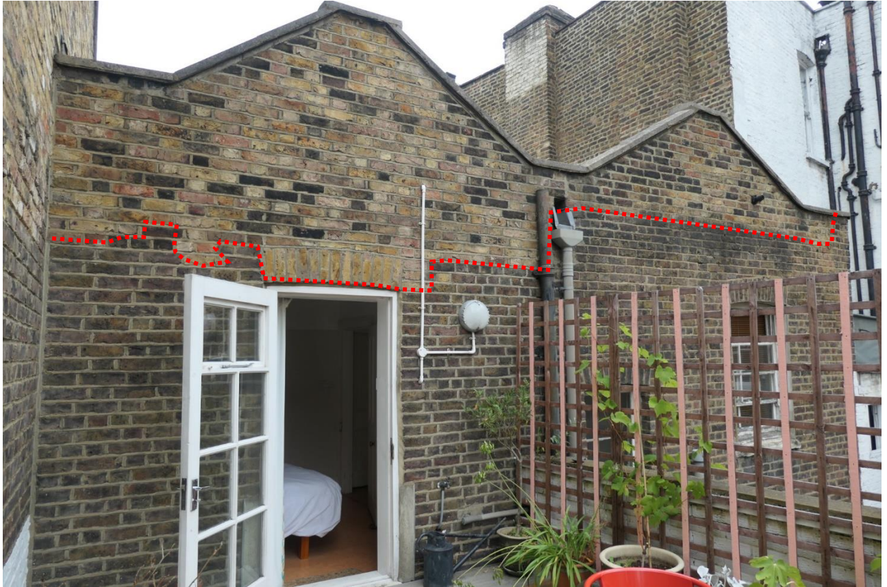
Photo 5: The rear gables, above the dotted red line, have been rebuilt.
