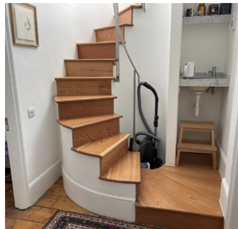
Stair to loft are not compliant with Building Control regulations
