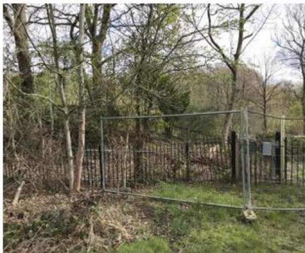
Existing low gate and railings at rear
