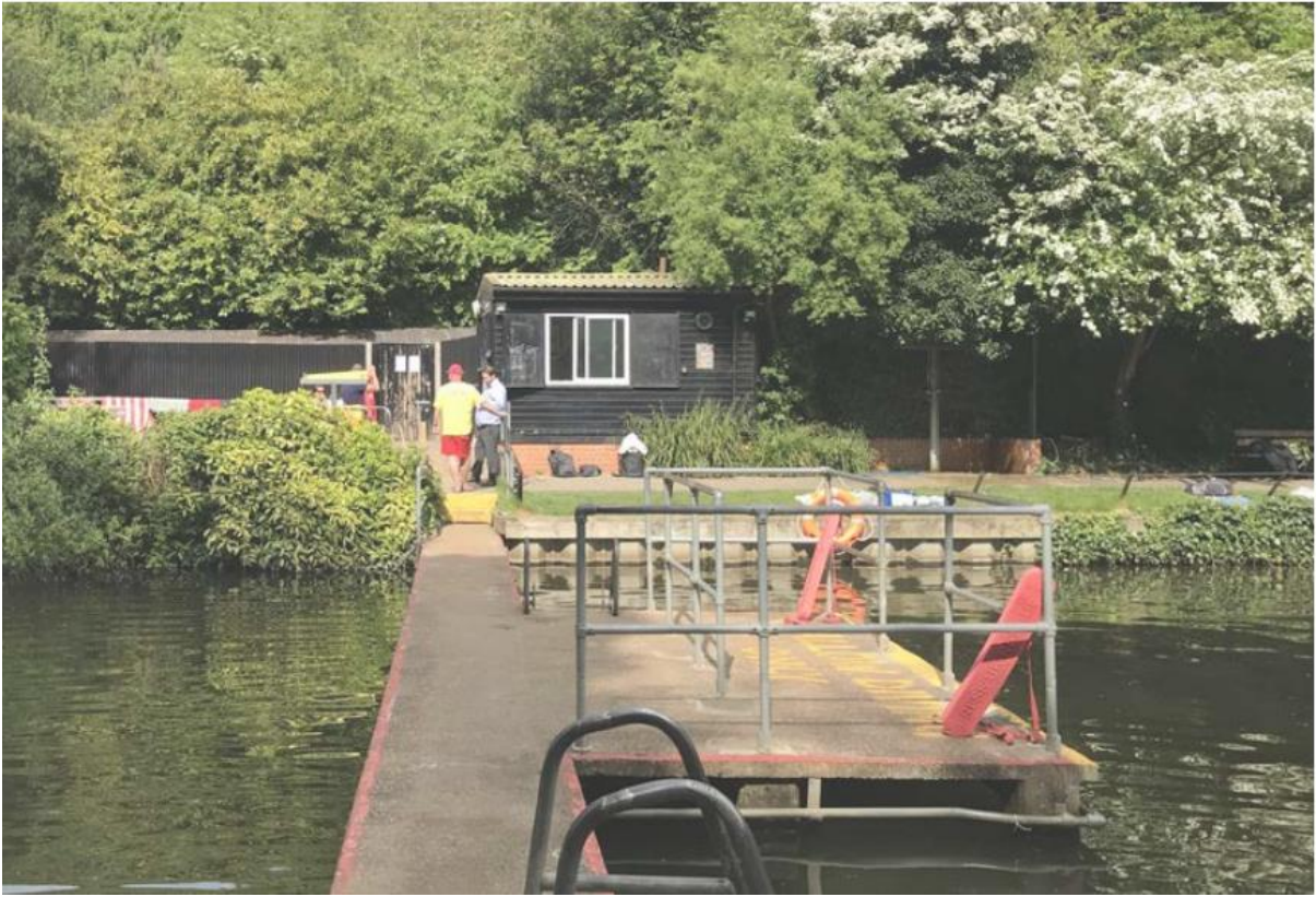
Lifeguard hut with changing rooms to rear
