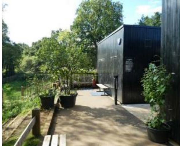
Existing timber clad changing/W.C. shower buildings
