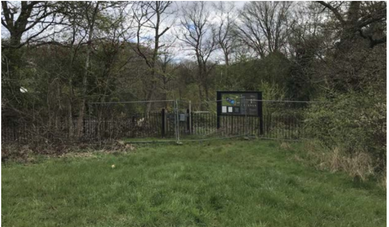
Existing low metal railings and temporary barriers – Ladies Pond
