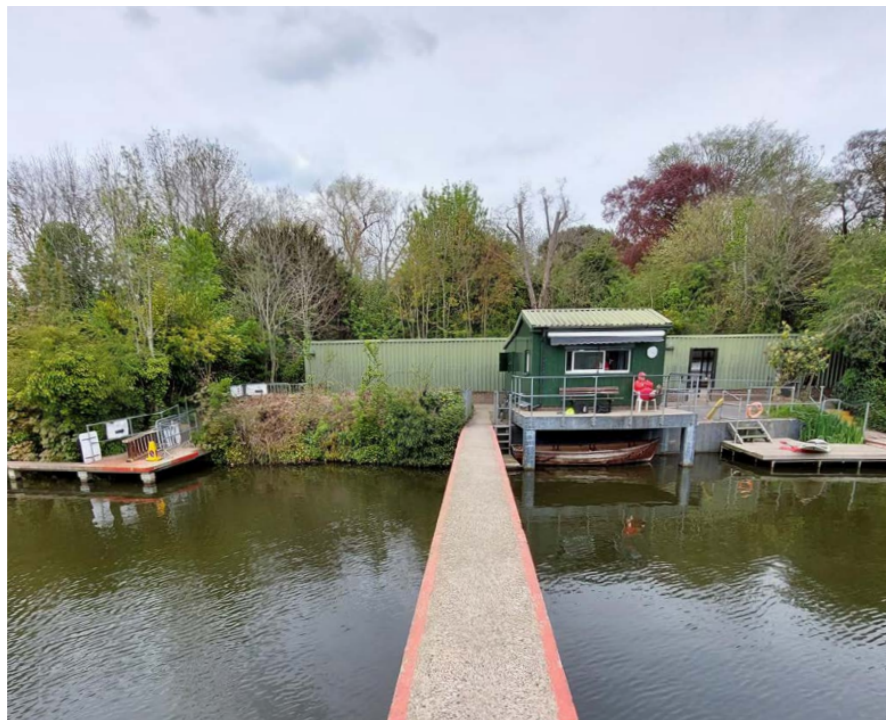
Existing changing rooms, walkways and lifeguard hut at Men's Pond
