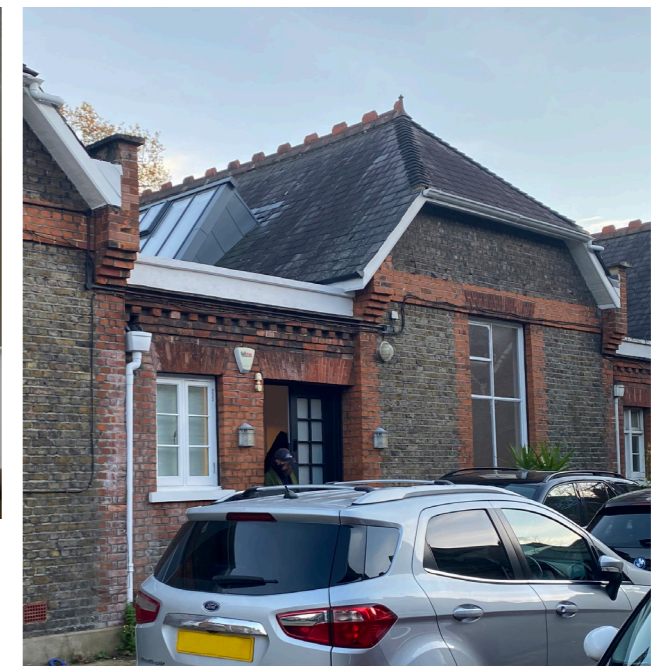
Site Photographs: Replacement rooflight at No.11 Primrose Hill Studios Approved Planning Application 2013/3740/P
