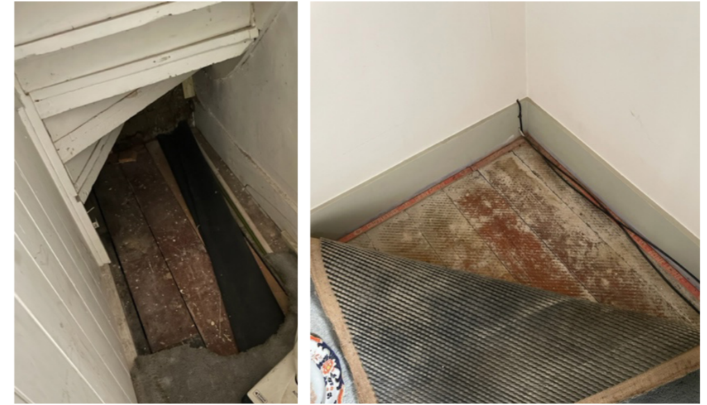
Existing timber floorboards in Studio 12
