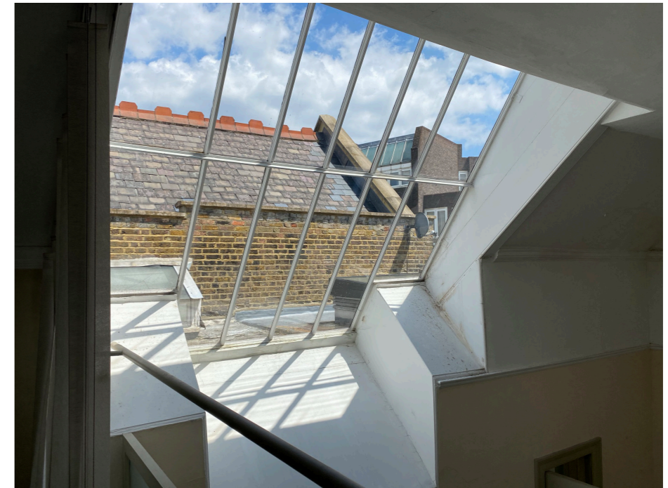
Site Photograph: Existing North Rooflight
