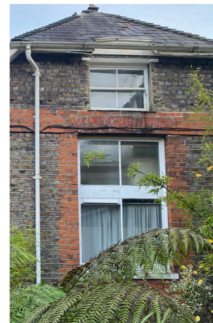
Existing west window
