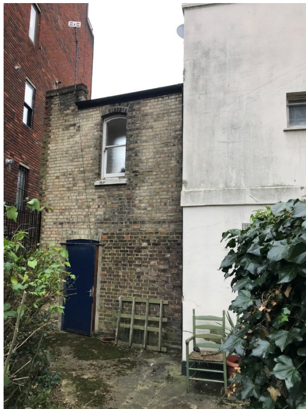
Side area looking at rear access
