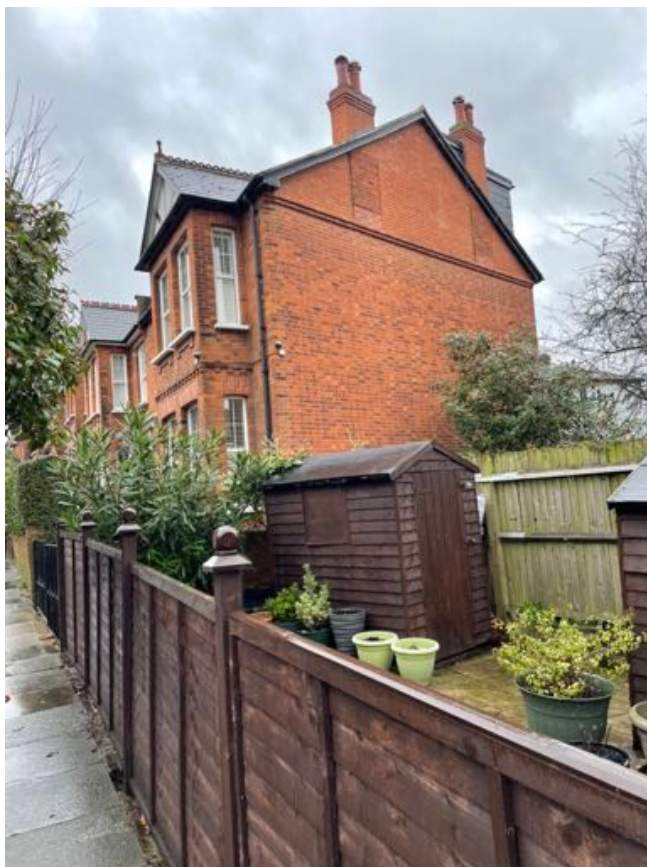
Gable Wall from St Gabriels Road
