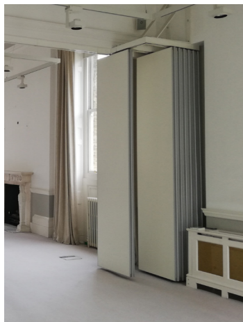
1 Non-original sliding false wall system in principle room, office R.1.02
