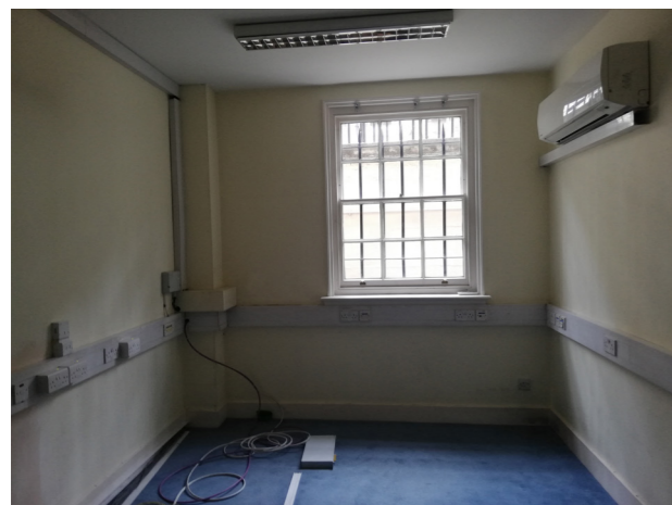
1 Existing condition of office, R.LG.12 illustrating existing face fixed cabling and electrics, and existing air conditioning unit
