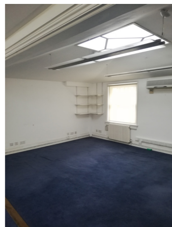
2 Existing rooflights in office R.2.09. Ceiling proposed to be removed and raised to existing roof line
