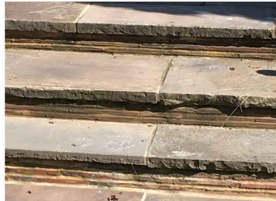
Steps with reclaimed York stone tread and tile creasing riser.
