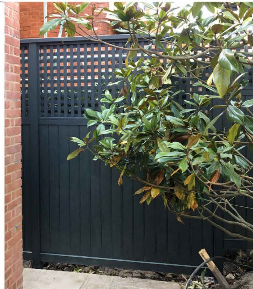
Timber fence with trellis at top, painted dark green.
