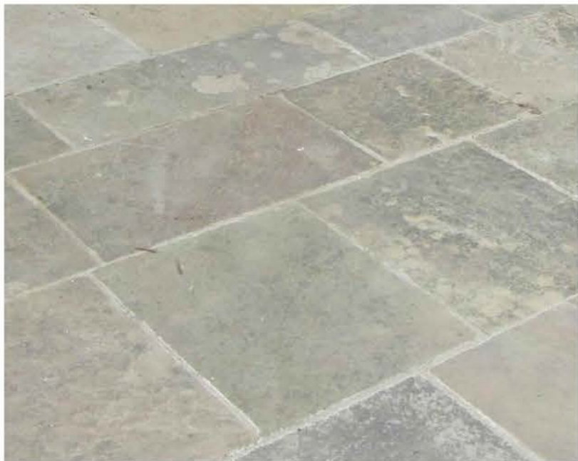
Reclaimed York stone paving with mortar joints.
