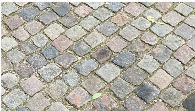
Granite setts with porous sand joints.
