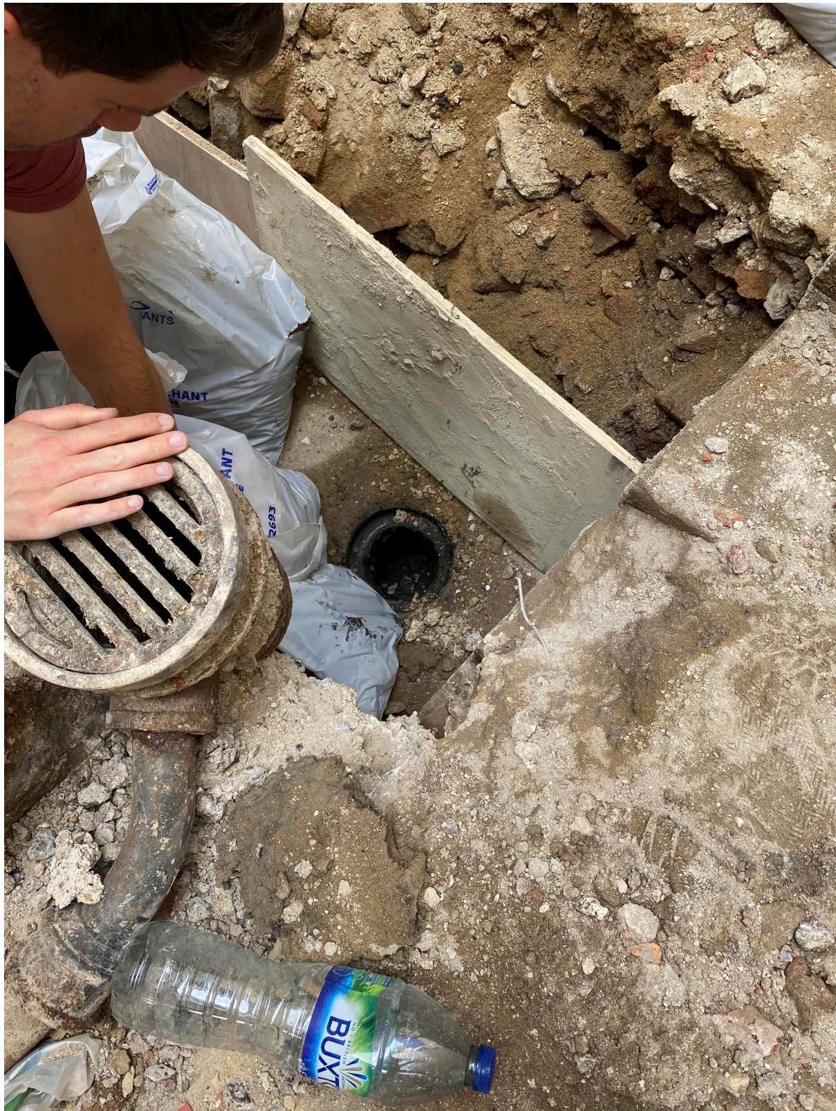
Photo 2: Original historic buried gully in comparison with non-original gully showing difference in level, with non-original back fill surrounding
