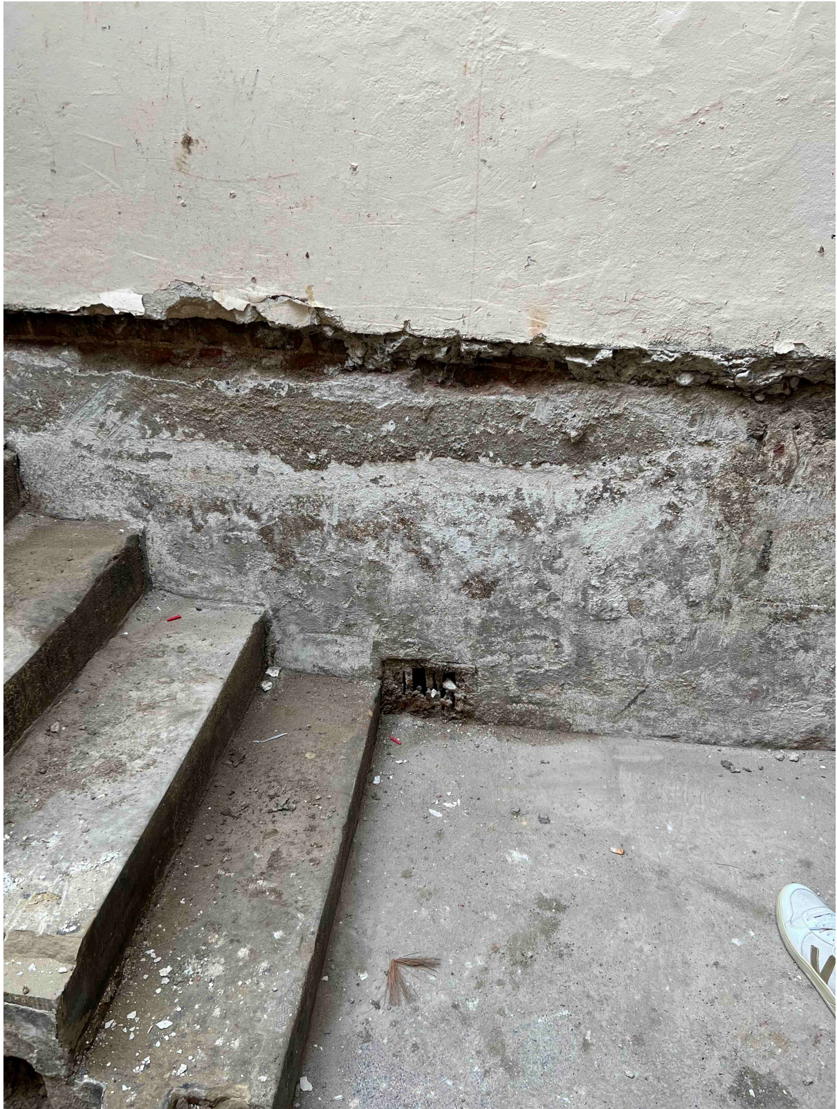
Photo 5: Original historic air brick located at bottom of the historic stair, showing that the original lightwell level was significantly lower than the existing
