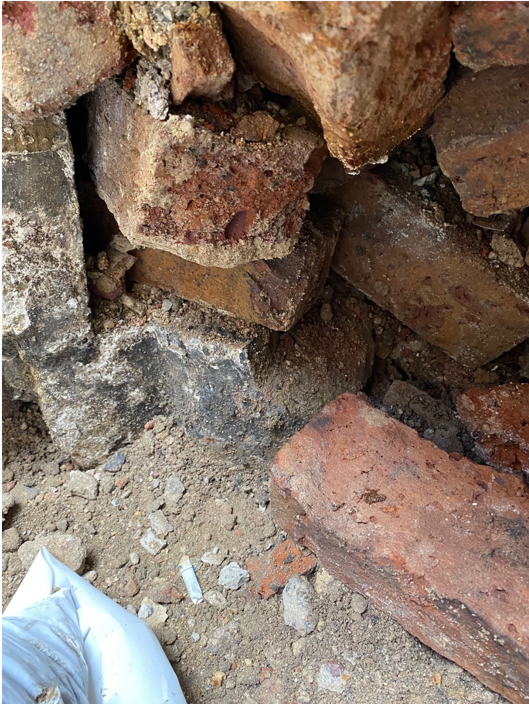
Photo 1: Original buried bottom step to existing stair, with non-original brick back fill
