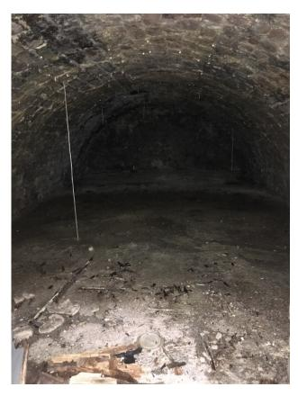
Three barrel vaulted cellars are under the pavement to the front of the property. All have replacement twentieth century doors, concrete floors and have been covered with a rough concrete render.
