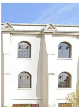
St. John's Downshire Hill
