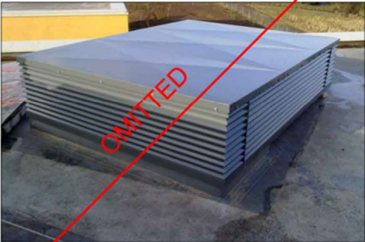
3 Louvered Penthouse Vent for AHU Exhaust
