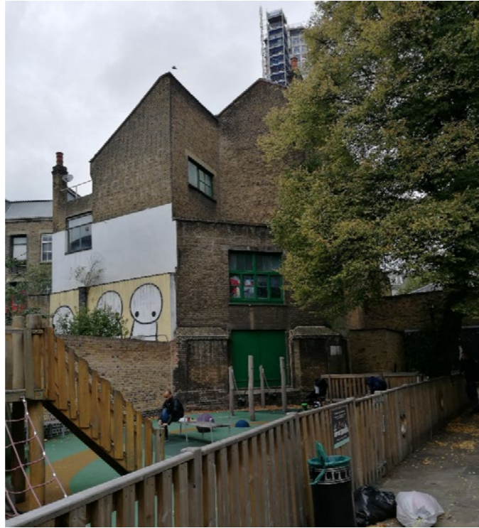
Figure 15: The rear of the building showing part of the original heptagon
