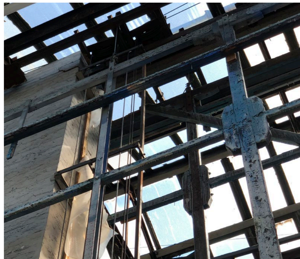
05 Existing condition of painting frames
