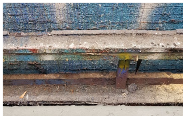
03 Existing condition of painting frames
