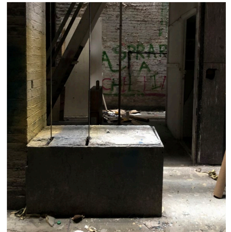
06 Winch to be retained and encased in clear box
