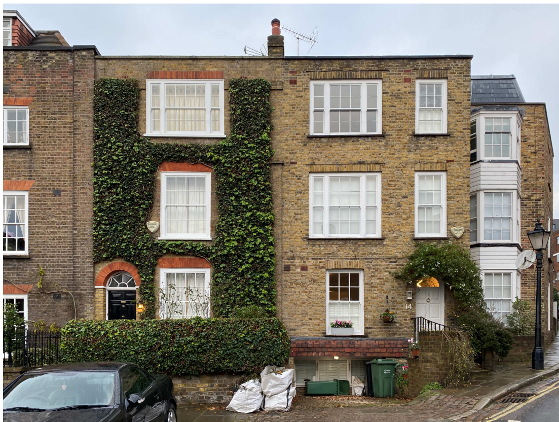
Above: photograph showing front façade. The brickwork is consistent across Nos. 14 and 16, being yellow stock brick seen elsewhere in the properties. Brickwork on the front façade is set in Flemish bond.
