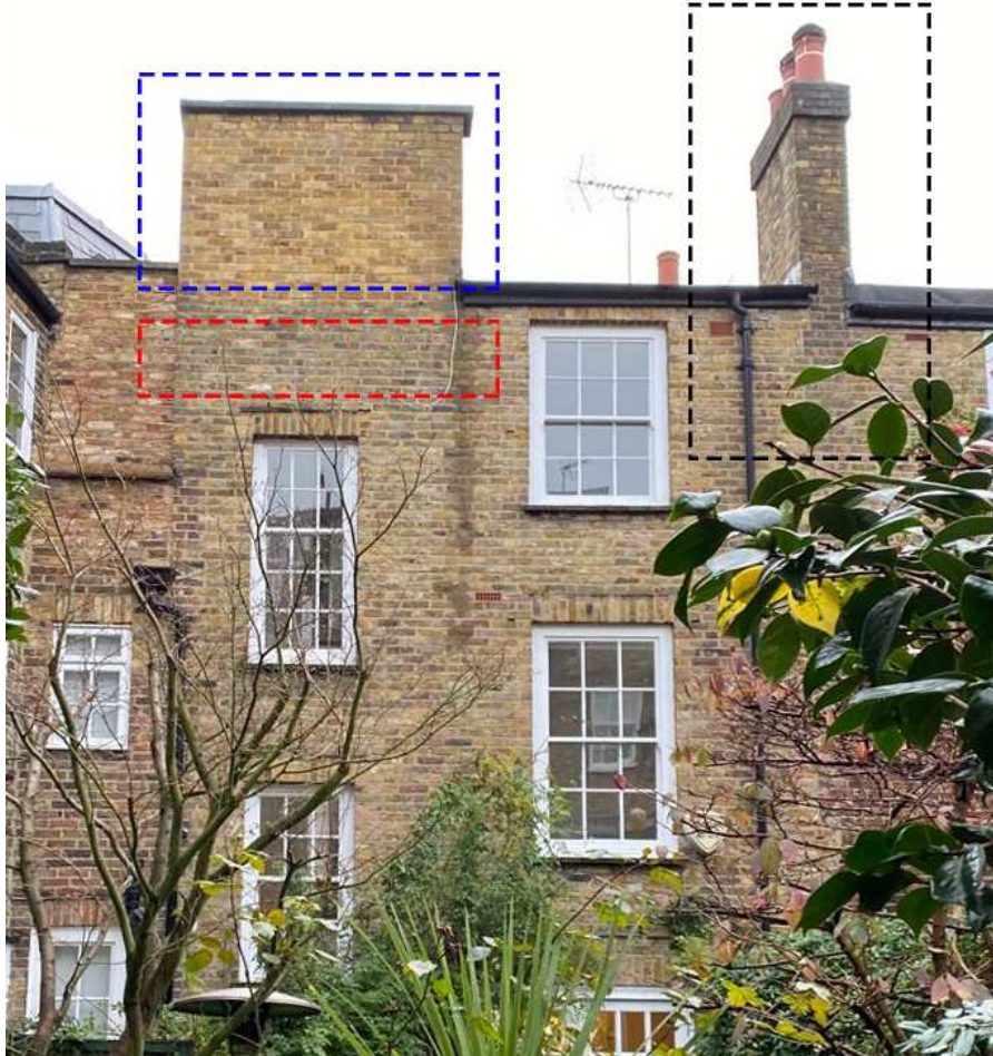
Above: photograph showing rear elevation of No. 14. Blue dashed area indicates newer, more yellow stock brick, in Stretcher bond, which is to be removed as part of the works. Red dashed area shows older stock brick, also in Stretcher Bond. Black dashed area indicates party wall adjoining No. 16, which is set in Flemish bond.
