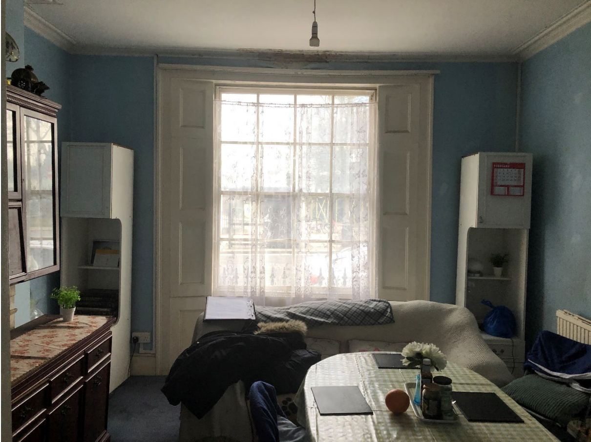
Figure 6 – Internal view of the timber sash window to the front of the building at ground floor level
