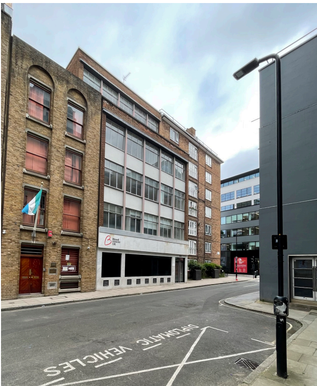
Above: Street View of 39 40 Eagle Street approaching from the West
