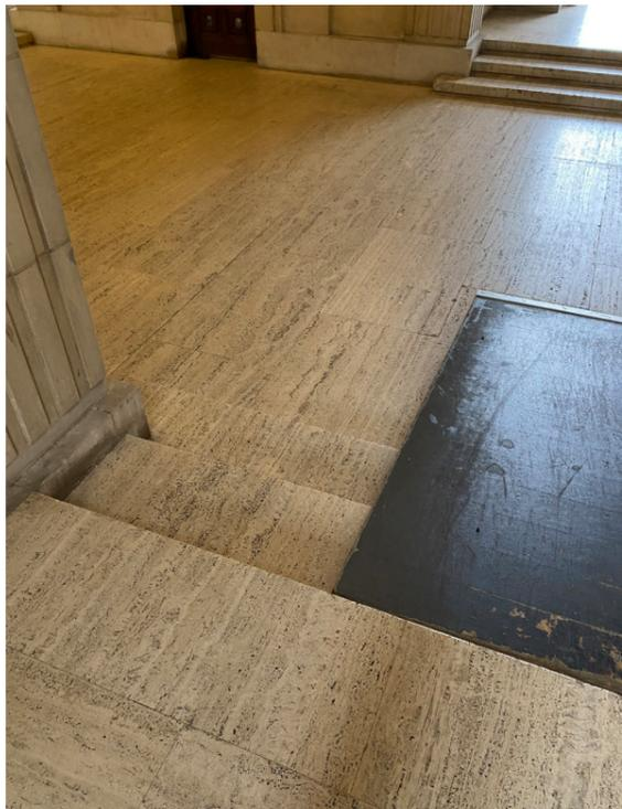
Figure 3.6 - Travertine Floor and temporary ramp example
