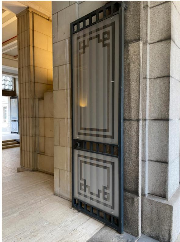
Figure 3.3 - Entrance Door featuring iron gate and perspex screen
