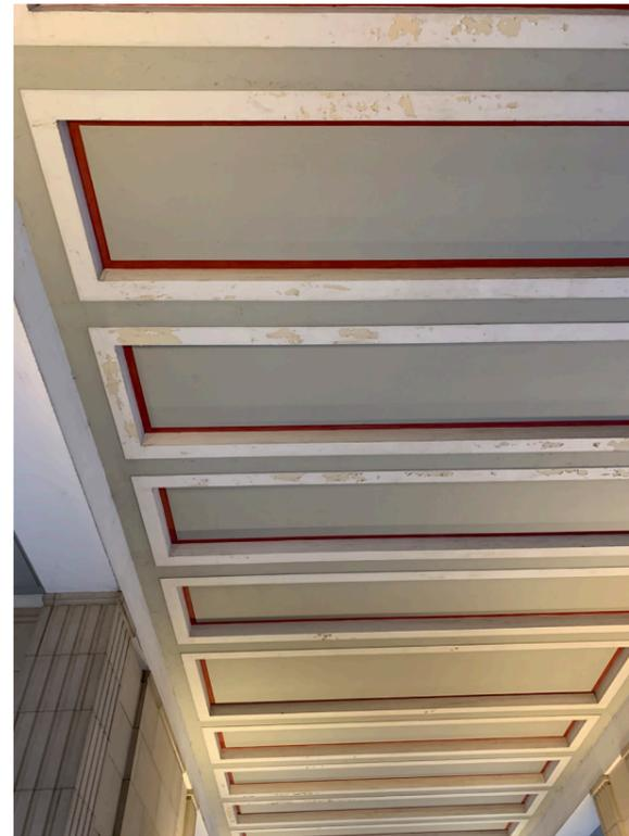
Figure 3.9 Ceiling details, showing signs of deterioration
