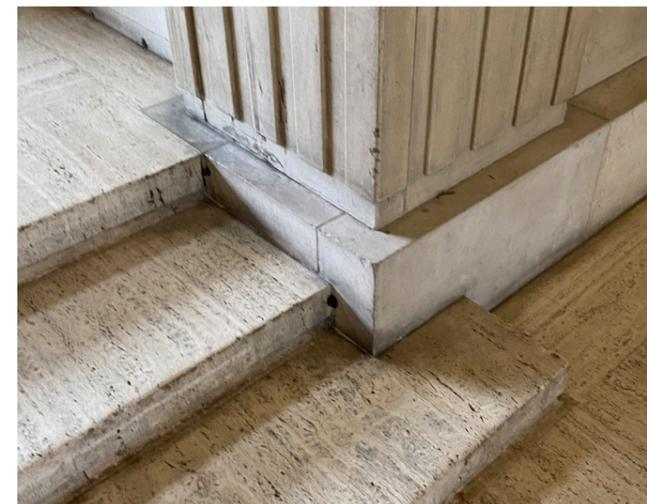
Figure 5.3 - Internal perimeter stair showing damage to travertine
