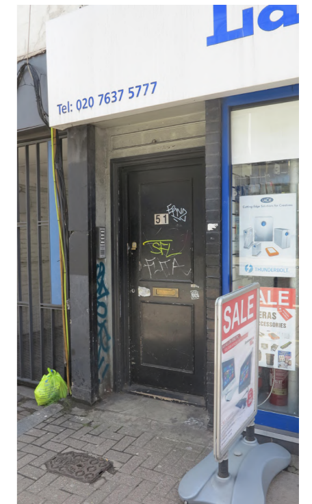
Fig: 2.35 Entrance to no. 51TCR
