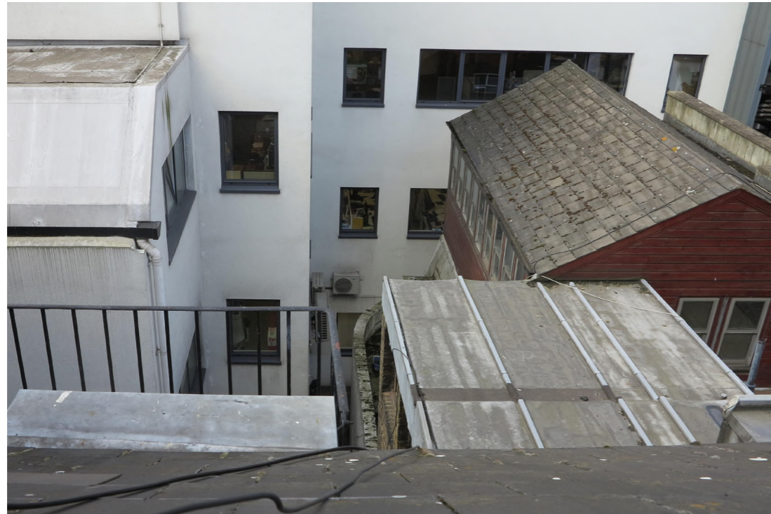
Fig: 2.36 View of rear roof no. 51 TCR
