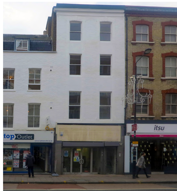
Fig: 2.27 No. 52TCR - Photo of Existing Elevation
