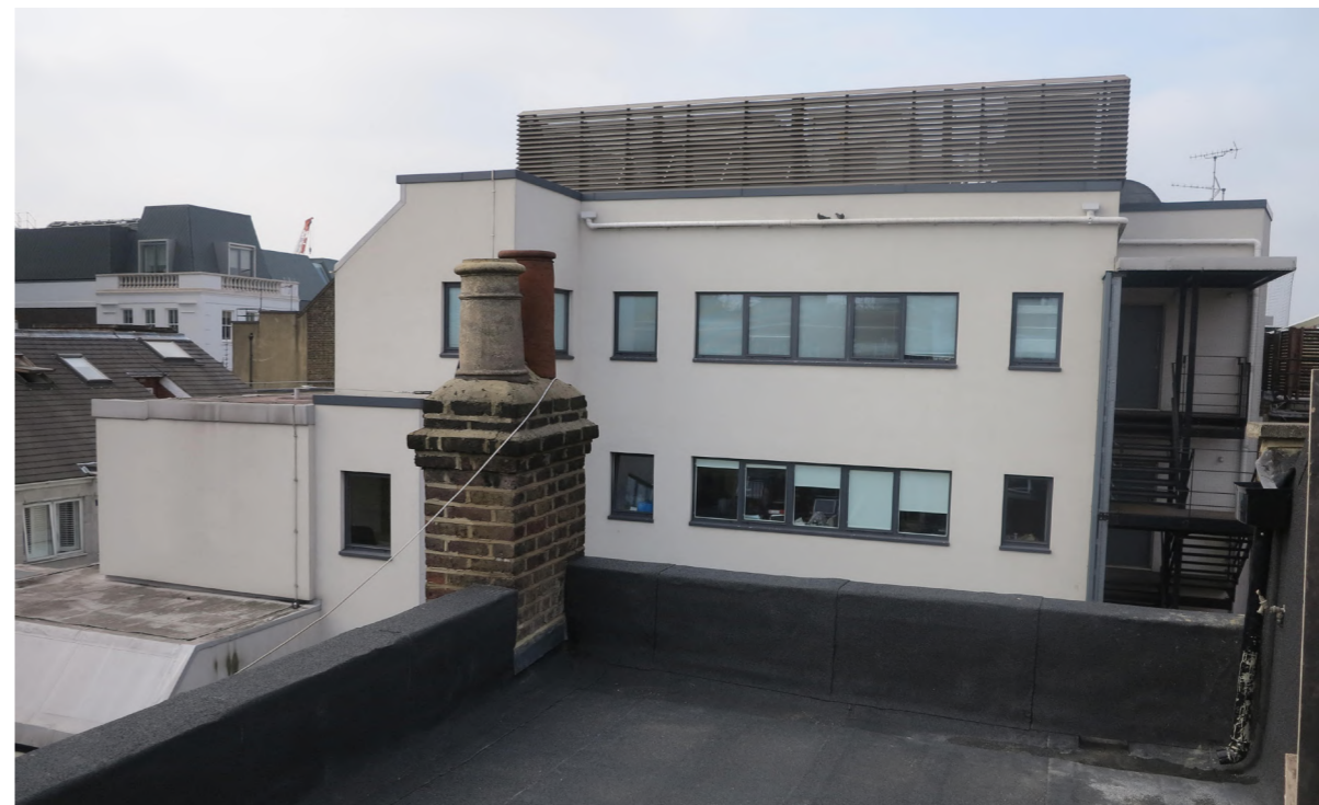
Fig: 2.39 View of rear 6-10 Whitfield St. Photo taken from roof of no. 52 TCR
