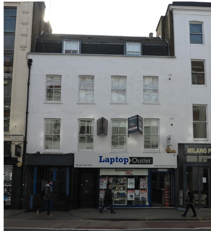
Fig: 2.25 No. 51TCR - Photo of Existing Elevation
