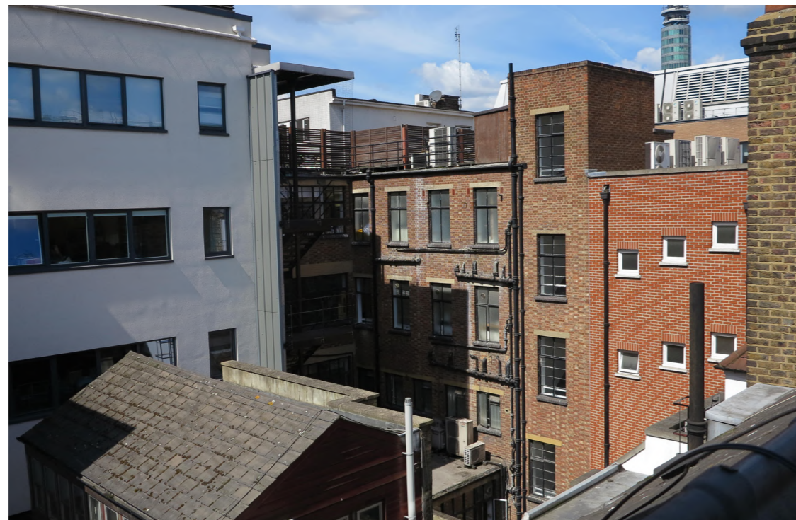
Fig: 2.38 View of rear roof no. 51 TCR, and rear elevations of buildings on Kirkman Place
