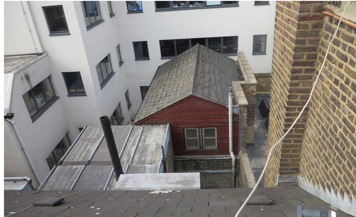
Fig: 2.37 View of rear roof no. 51 - 52 TCR
