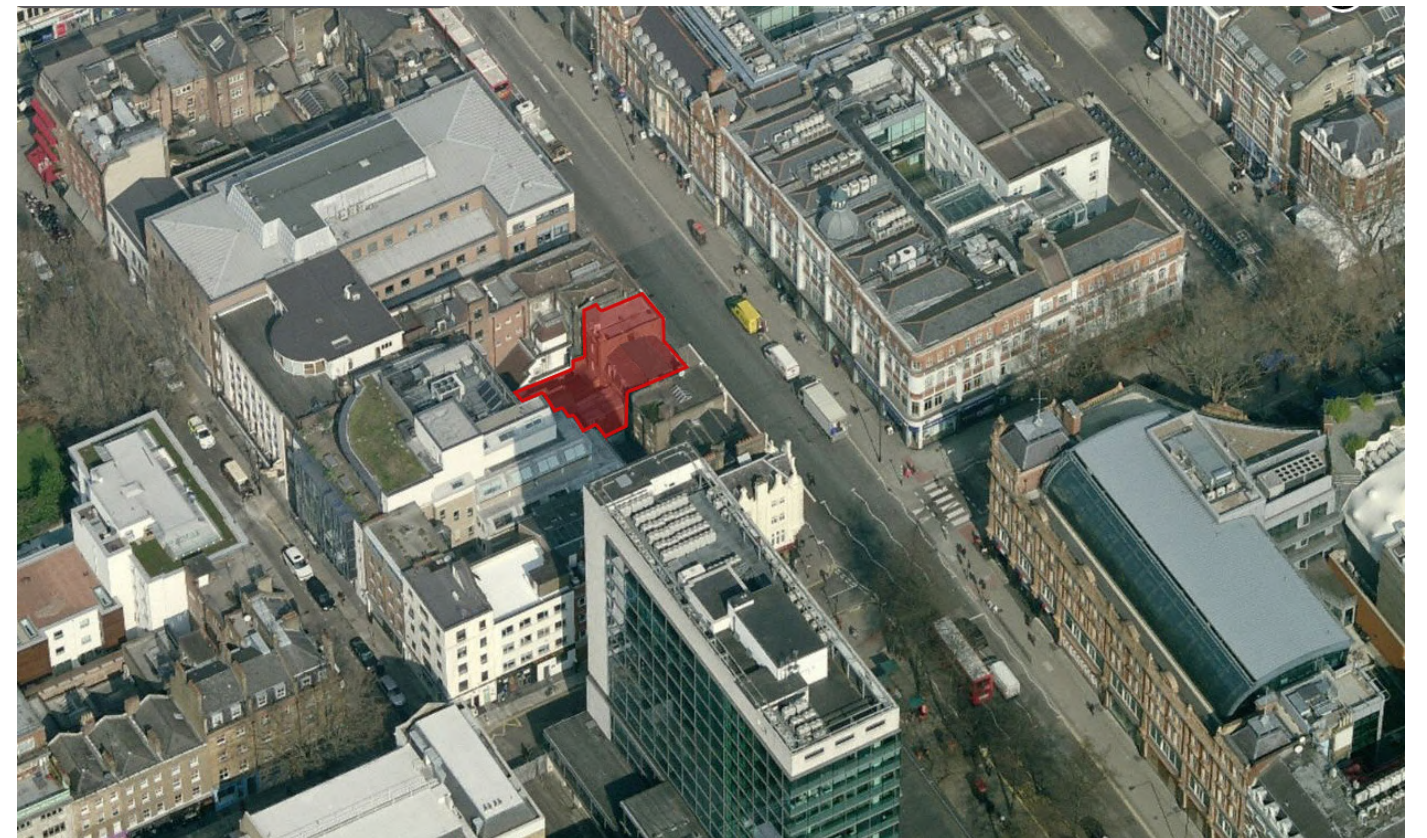
Fig: 2.10 Aerial Photograph from south
