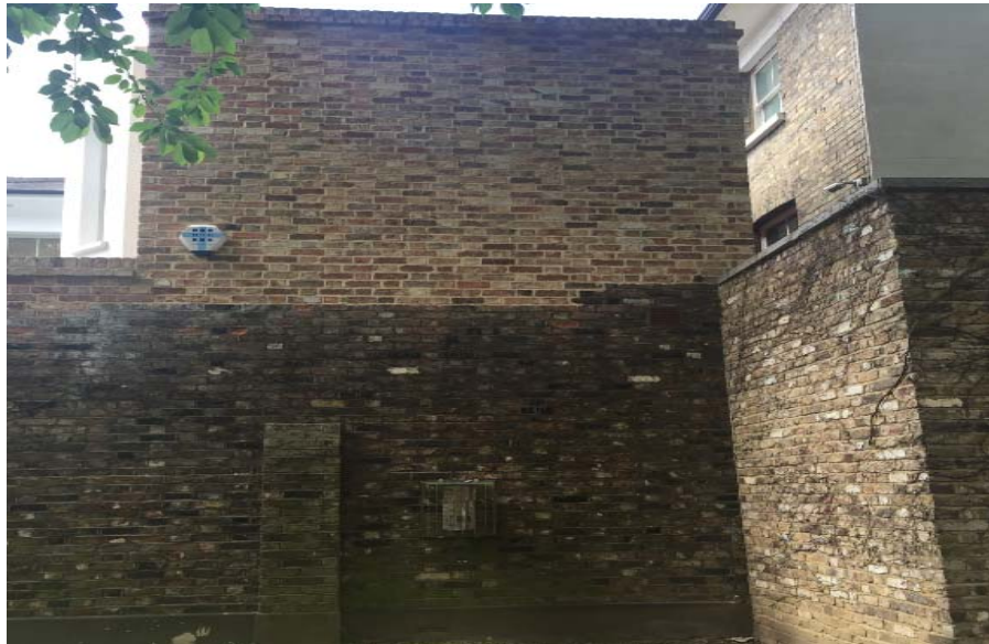
Figure 13: 37 Greville Road - rear (north) elevation
