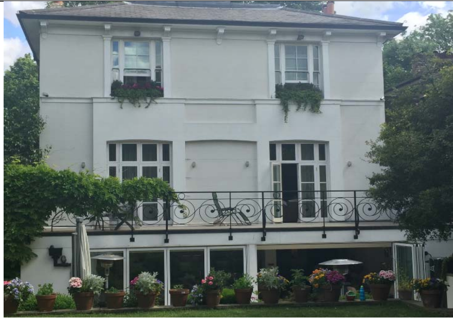
Figure 1: Side elevation, viewed from South-west
