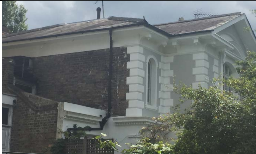
Figure 12: 37 Greville Road front/side corner elevation
