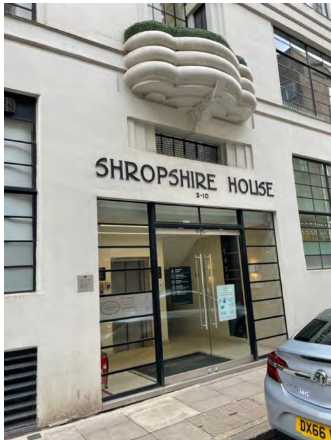
3.1.C Photo of Existing Main Entrance Door
