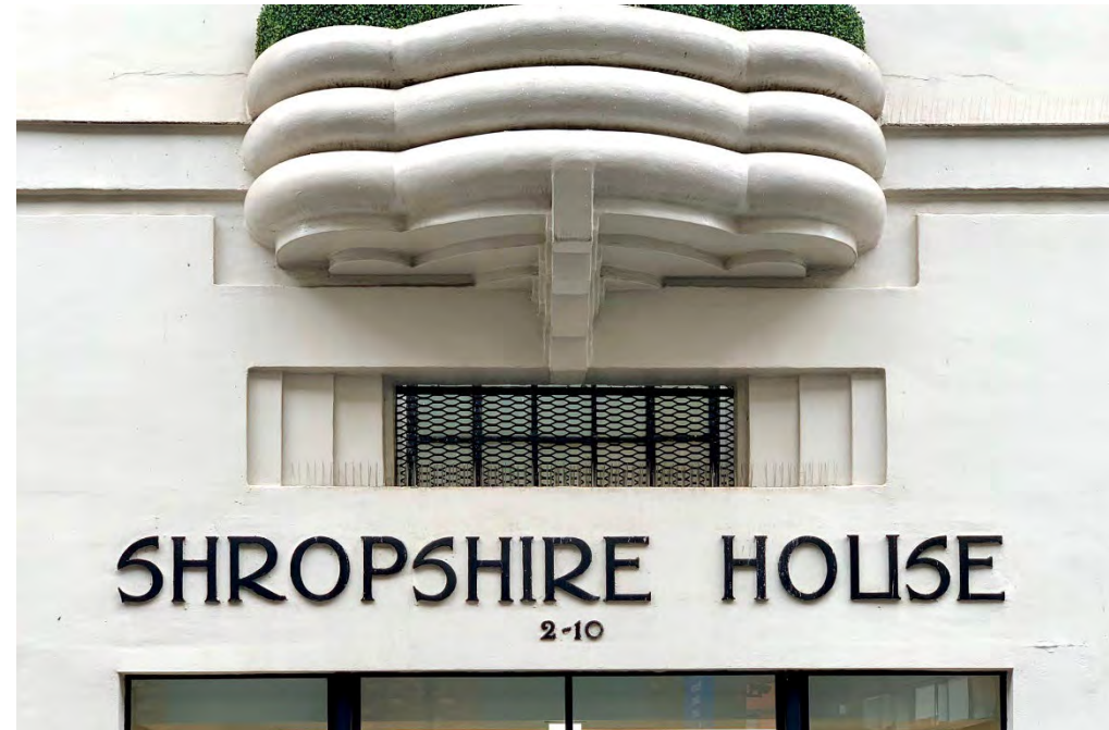
6.1.b Existing Photos of Building Numbers (West Entrance)
