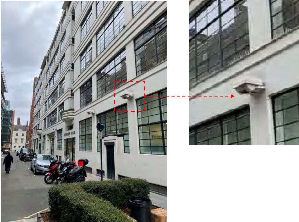
5.1.A. Existing Front Elevation down-lighters
