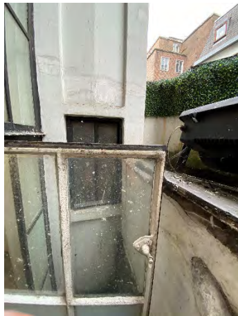
2.1.E: Image of Glazing to side reveals of front feature alcoves – Capper Street
