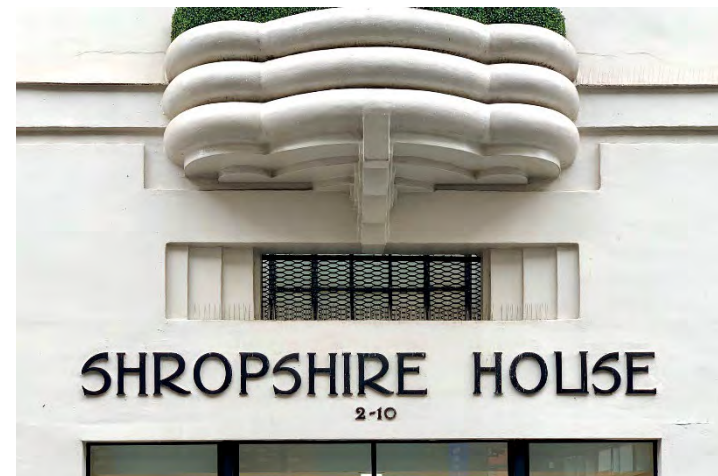
6.1.D: Use existing recess detail to fix new 'building number' signage. Note; refer to HHD dwg no. 256.400.01/ 256.400.02 & 256.401)
