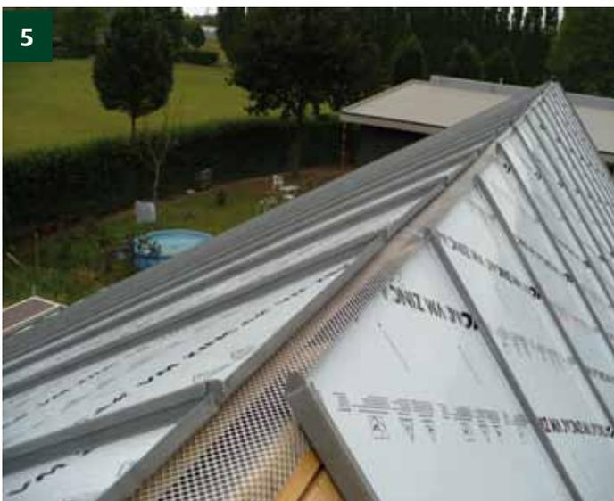
In the case of a vented roof, between the last boarding planks of each roof pitch provide a ventilation opening, protected by the insect mesh, (minimum 35 mm). The space between the Standing seam trays on the each side of the roof must be 30 mm wide.
