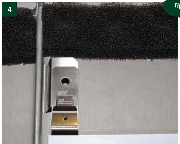
The placement of the clip is easy; it should not be twisted into the Standing seam. The position of the clip may be easily adjusted by sliding it upwards or downwards. If necessary use a bevelled nylon or wooden mallet. Take care that the clip G3 has not been twisted or has not been poorly placed in the Standing seam or been damaged.
