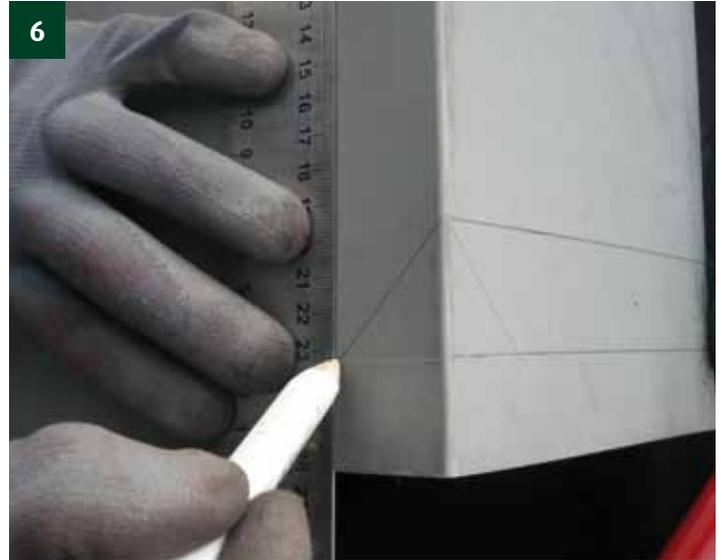
At the intersection of the diagonal line (half angle of the roof) and the 30 mm line, draw a perpendicular line to the edge of the ridge element.
