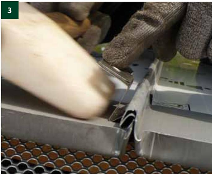
Place the clips G3 on both roof inclines. Place the underside of the clips on the line of the cut-off of the film. Manually slide the clip into the Standing seam without opening the Standing seam.
