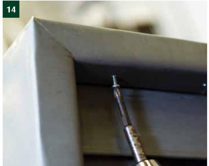
Fasten the ridge G3 element into the verge edge with a stainless steel screw. Do this on each side.
