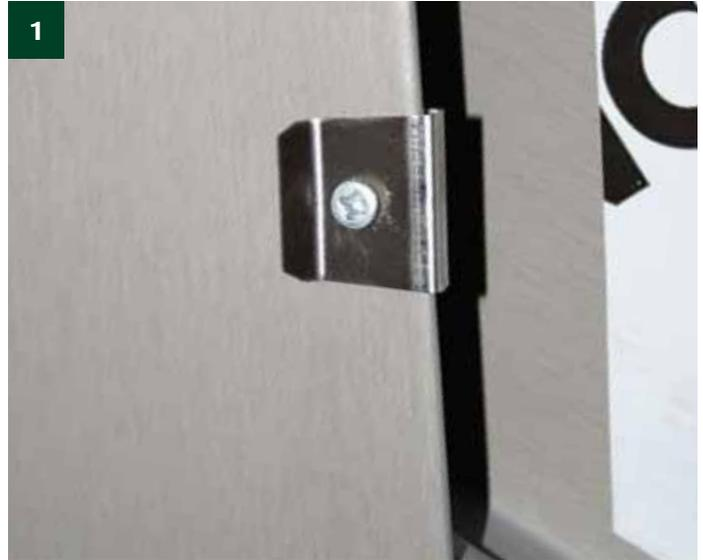
In order to prevent the G3 Hip element from sliding away, a stainless steel screw (self-tapping stainless steel Type SPS 3-7,1-4,5x18mm) is screwed into each clip. Use a bit number SR 1.
