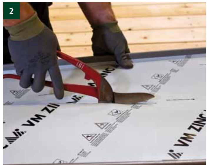
Connecting the verge trays. The preparation: cut the outside of Standing seam tray, on the visible width (minimum 150 mm and maximum 370 mm) + 35 mm.
