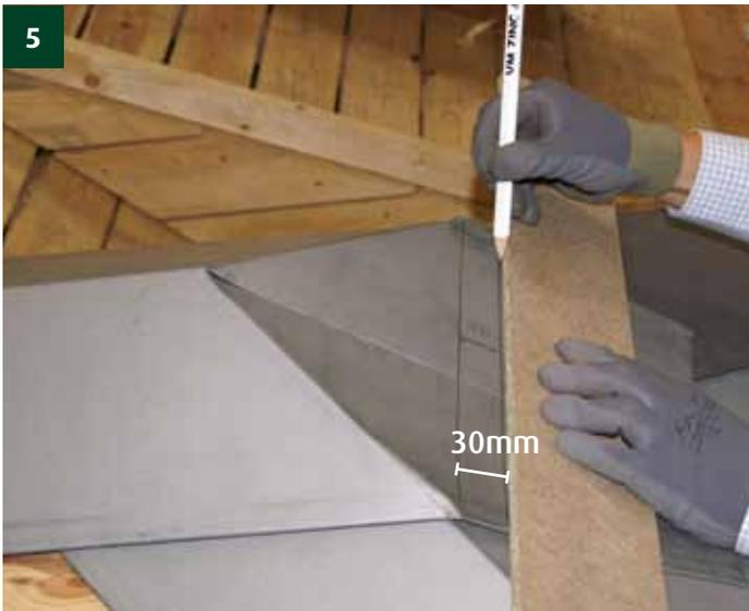
Place the ridge element on the roof, trace a horizontal line 30 mm below the edge of the ridge element.
