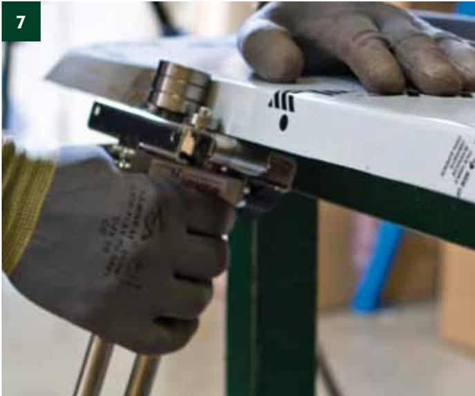
After the placement of the Standing seam trays on the Verge G3, one folds the overhanging outside edge over the nose of the eaves apron strip G3. Finally, close the prepared fold around the eaves apron strip G3 with flat folding pincers.
