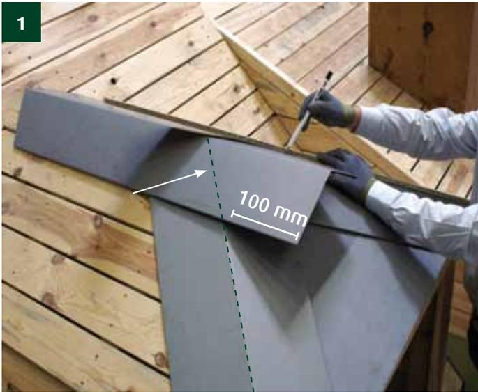
1 Cut the ridge G3 (length that's needed + 100mm over the ends) Place the ridge G3 element without fixing it Trace on both sides a line on the crossing between the hip and the ridge G3 element.
