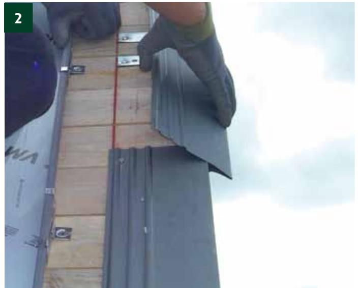
2 Hook the verge strip firmly into the sheet clips and nail them firmly just as you did for the eave. The elements overlap each other by 50 mm. Place the verge G3 from bottom to top.
