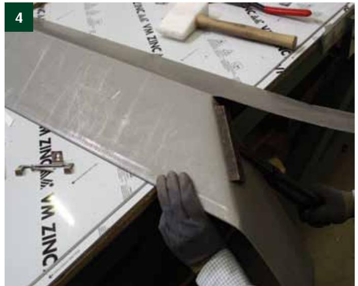
4 Fold both sides of the element, use the lines as the indicator on where to fold, take also the pitch into consideration.
