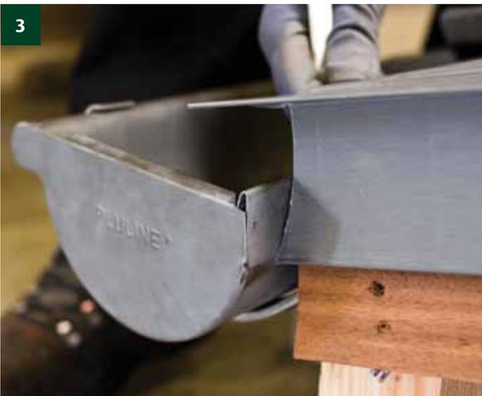
3 In order to obtain a perfect aesthetic result we recommend you to first fold the eaves apron strip at 90°. The drip of the first verge G3 (at each interior angle of the roof) is cut off at the bottom, in order to fit into the profile of the gutter used.
