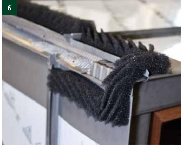
Press the decompression strips properly against each other (maximum 1 joint per Standing seam width) in order to ensure a continuous weather tightness. The VMZINC® must be dry and free from dust before the decompression strips are mounted. Please ensure the continuity of decompression strip on the ridge ends.
