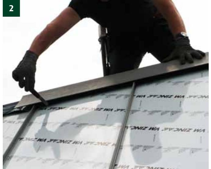
By means of a ridge element, that has been correctly mounted on the axis of the roof, but has not yet been fastened: mark and remove the protective film on both sides of the ridge, at the head of the Standing seam trays, using a sliding blade utility knife (without damaging the zinc).
