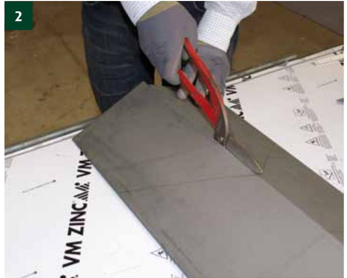
2 Cut the centre line of the hip element, upto the intersection of the 2 other lines.
