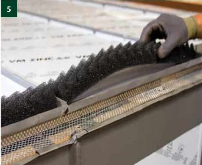
Stick the decompression strip onto the Standing seam panel, just above the clips (minimum 10 mm from 15 mm upstand). Length of each decompression strip = width of the strip + 20 mm. It is permissible to recover the leftovers, which have a minimum length of 150 mm.
