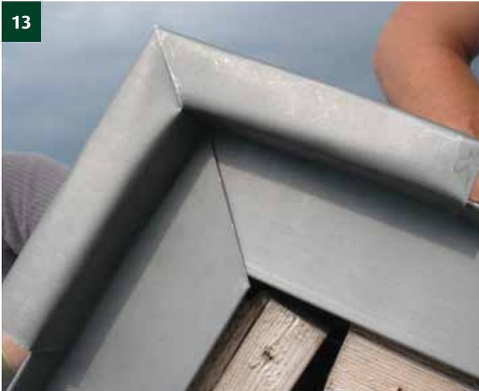
Position the last ridge element by hooking the fold back in under the Verge G3.
