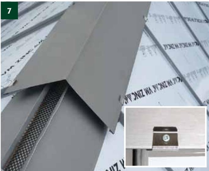
Adjust the angle of the ridge cap using a folding machine/angle bending machine in proportion to the roof incline and then click it firmly into each of the clip (you should hear a click). In one movement screw in and properly tighten a stainless steel screw type SPS 3-7,1-4.5 x 18mm from SFS or equivalent. Use a number SR1 bit for this.
