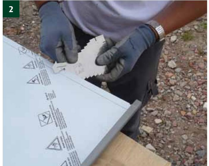
2 For the realization of the head: trace the strip on 15 mm.
