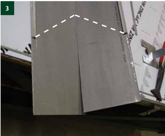
3 Cut away the folds on both sides upto the drawn lines.
