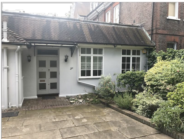
Existing Entrance Door
