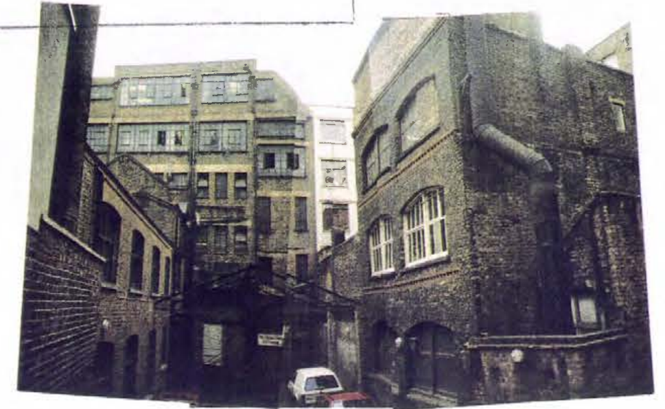
View from rear of number 4 Flitcroft Street
