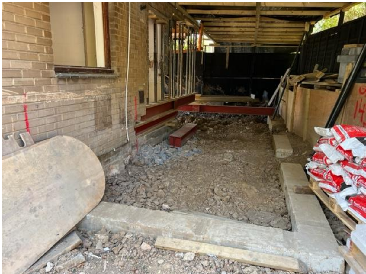
SITE PHOTOS SHOWING FOUNDATIONS FOR SIDE AND REAR EXTENSIONS IN PLACE AND STEELWORK MODIFICATIONS TO GROUND FLOOR UNDER WAY
