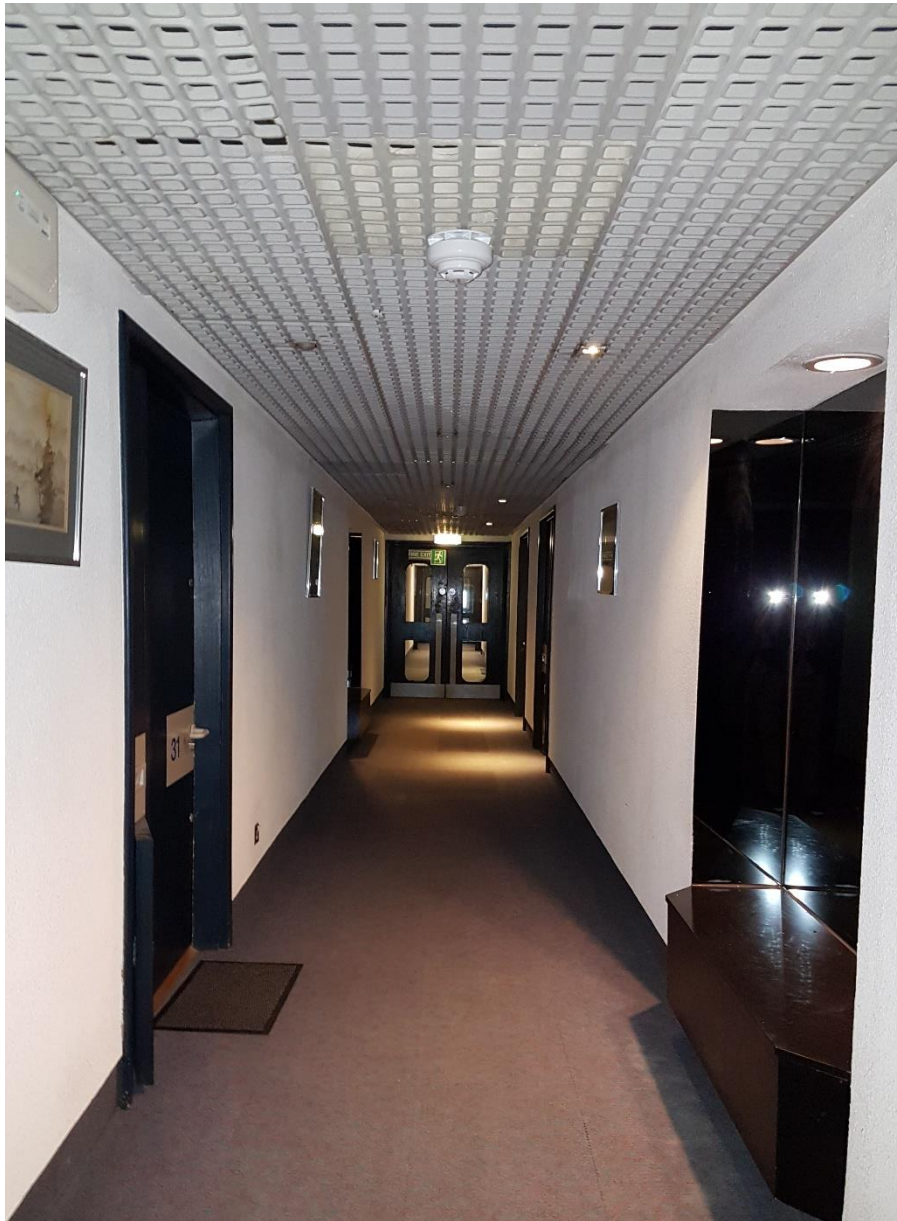
Photograph 8: Typical view of existing suspended ceiling and inadequate lighting to corridors
