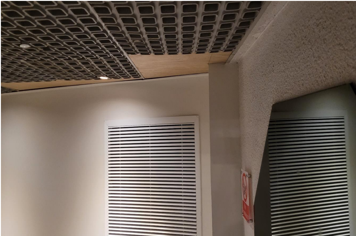
Photograph 3: Typical plywood sheeting to 5 th floor lift lobby ceiling where ceiling tiles missing
