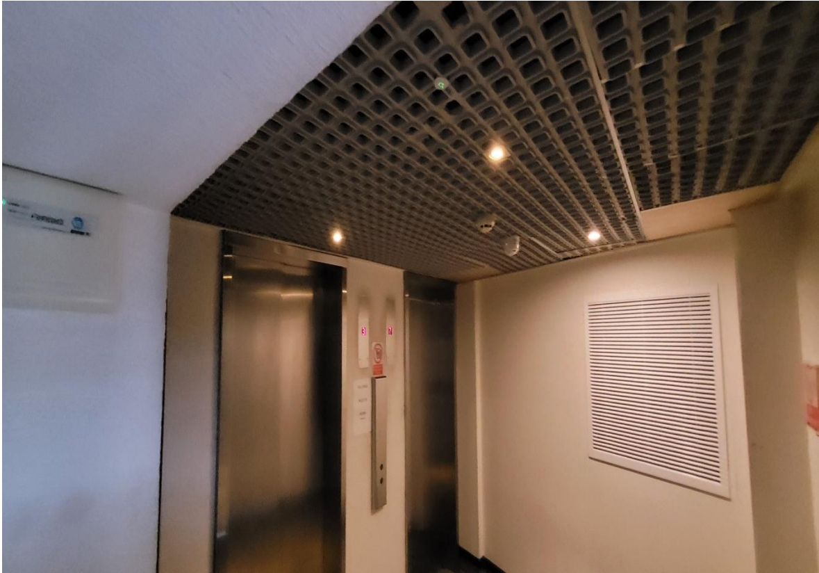
Photograph 1: Typical plywood sheeting to 3 rd floor lift lobby ceiling where ceiling tiles missing
