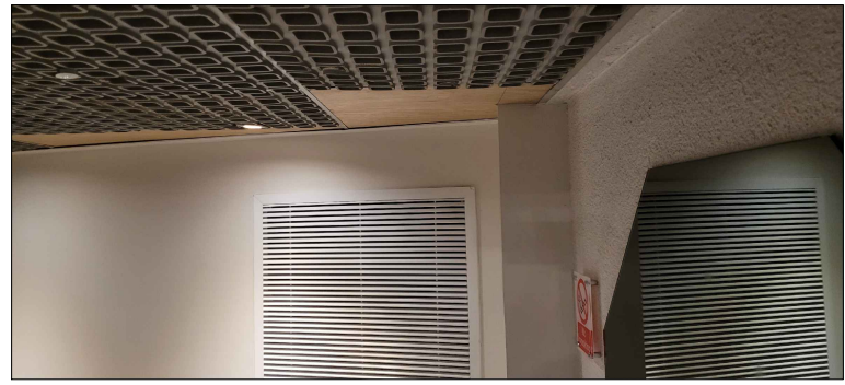
Plywood sheets where suspended ceiling tiles missing/ damaged in lift lobby
