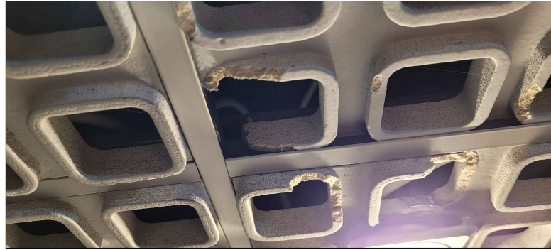
Typical damage to existing ceiling tiles
