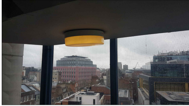
Existing Light Fittings Type (B) Basic 2D circular bulkhead light fittings surface mounted to ceilings throughout staircases.
