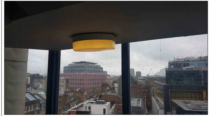
Existing Light Fittings Type (B) Basic 2D circular bulkhead light fittings surface mounted to ceilings throughout staircases.
