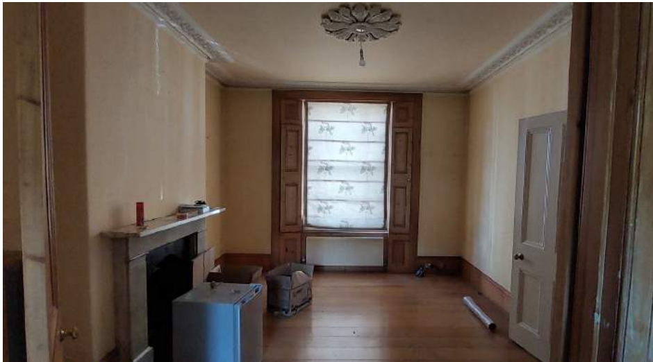
Original timber panelling, ornate cornice details and ceiling rose
