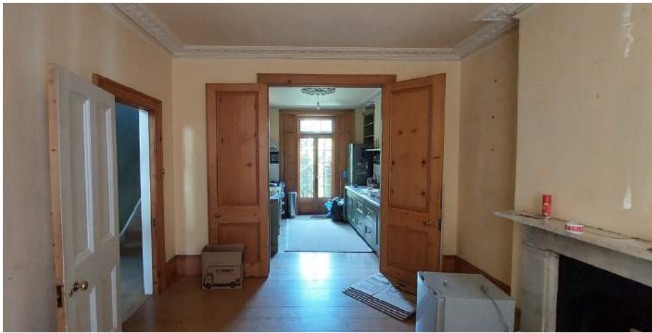
Original timber panelling, ornate cornice details and ceiling rose
