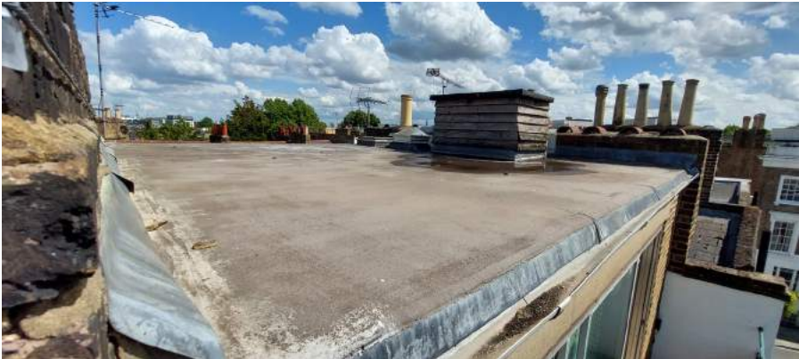
Asphalt roof and edge conditions, and water tank enclosure
