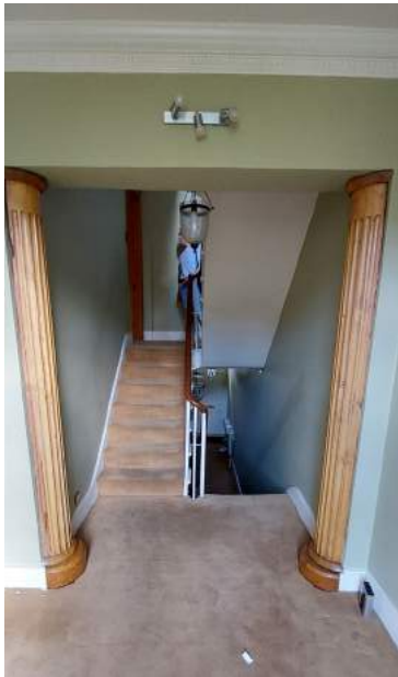
Non-original timber column additions
