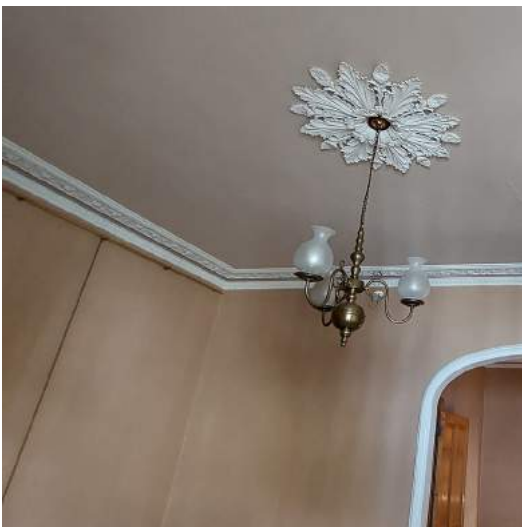
Original ceiling rose and cornice details
