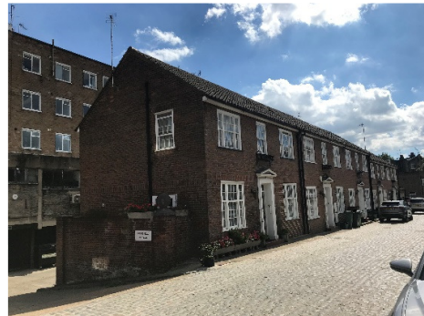
EXISTING STREET VIEW
