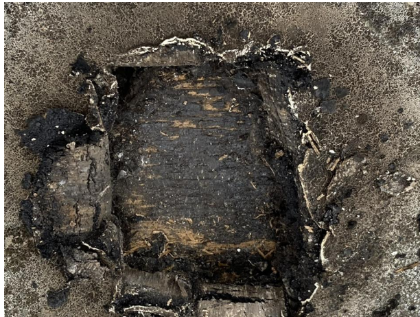
Asphalt on close boarded timber.
