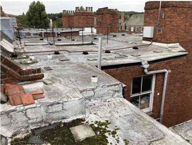
Overview of typical main roof area.
