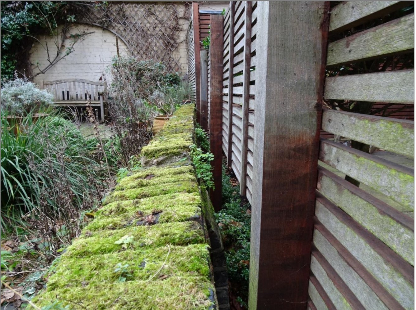
Photograph 6 Party fence wall with 37 Gloucester Crescent.
