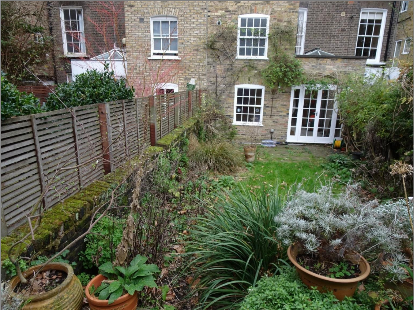
Photograph 5 Party fence wall with 37 Gloucester Crescent.
