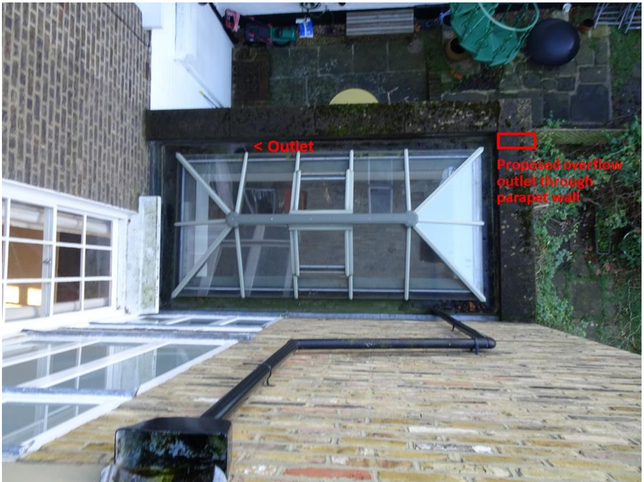
Photograph 2 Conservatory extension roof.
