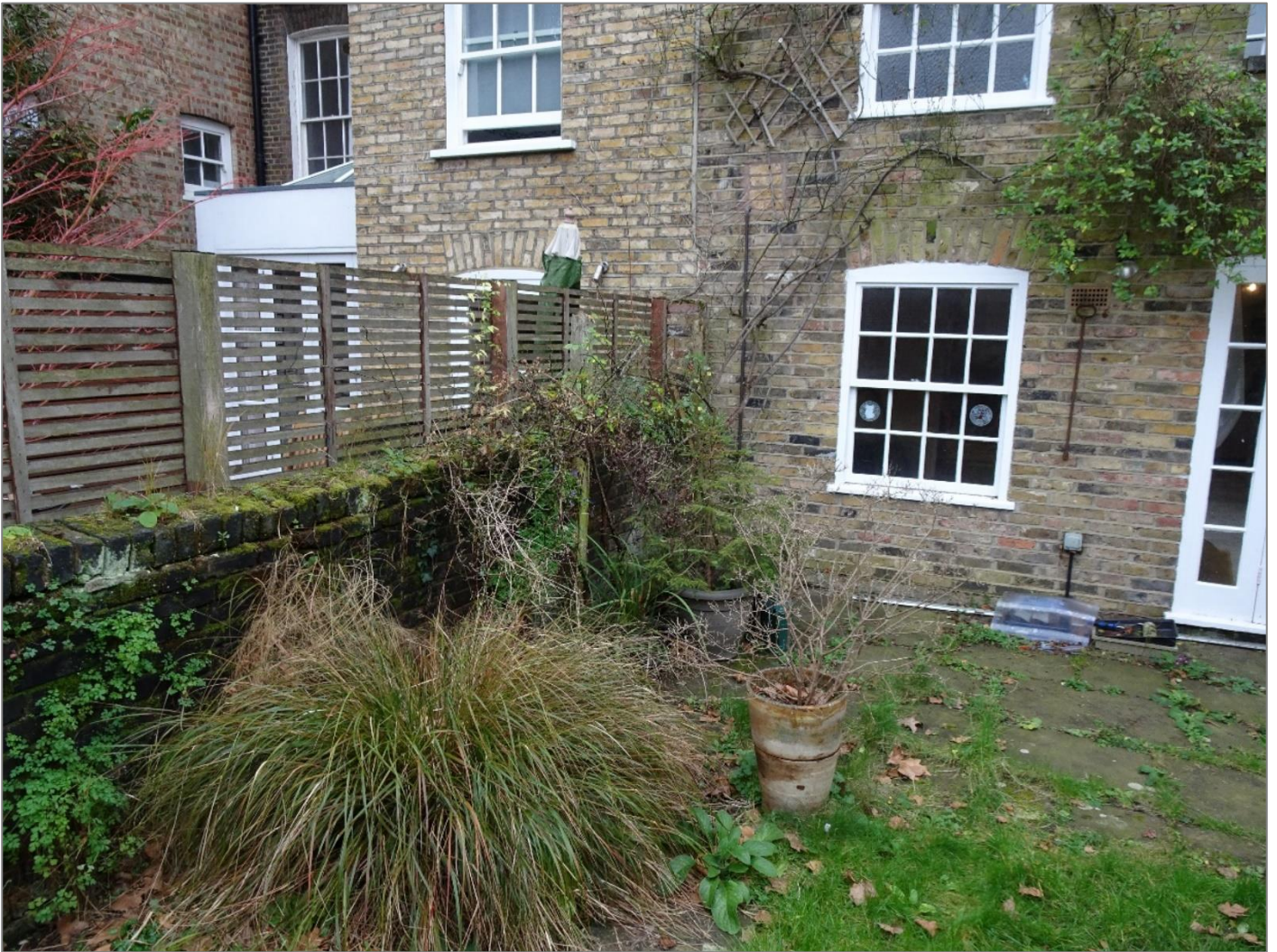
Photograph 7 Party fence wall with 37 Gloucester Crescent.
