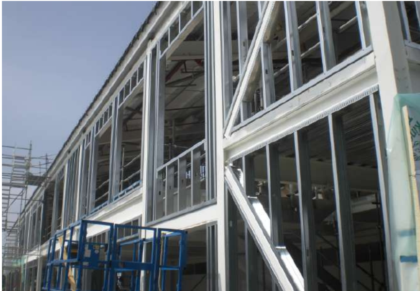
Photo 1: Example of hot rolled frame structure with light weight metsec wall infill and floors.
