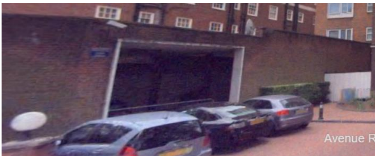
Figure 10 – Existing Ground Floor ancillary area
