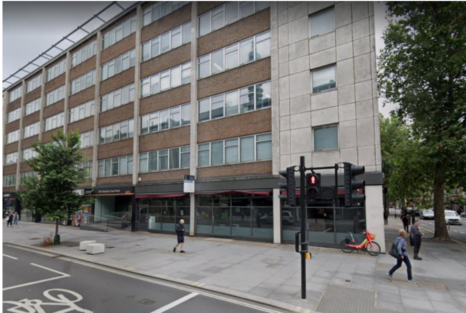
Figure 2: Existing unit (Source: Google Street View)
