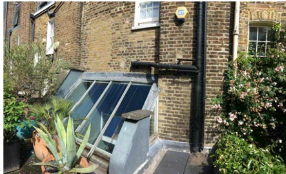
roof terrace & sloping glazing
