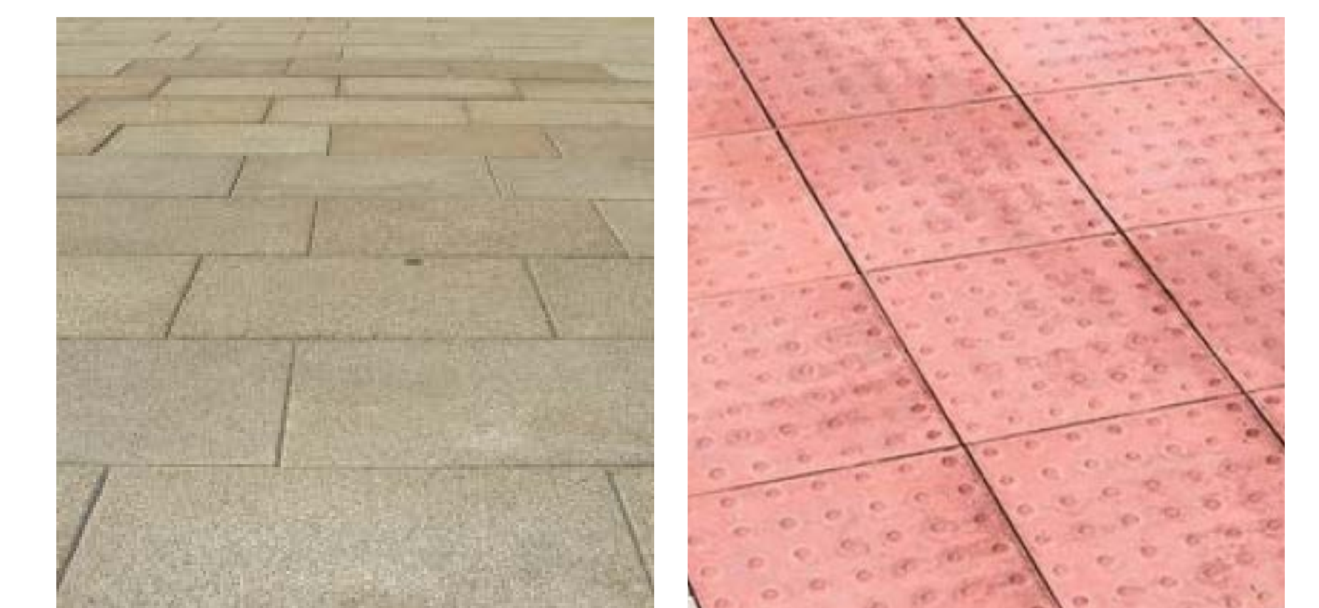
ASP flag paving to existing footways
