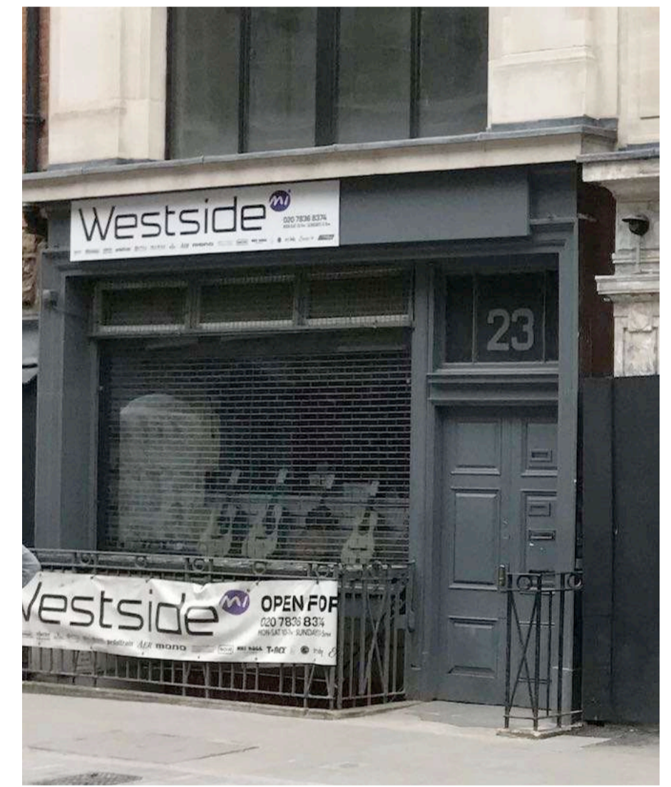
5 Existing shopfront to 23 Denmark St Scale: 1:50
