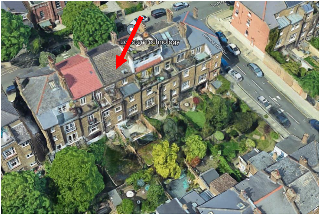
Application site marked with red arrow
