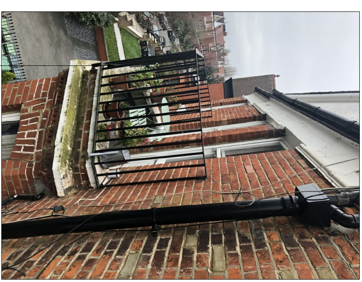
EXISTING NEIGHBOUR'S BALCONY - PHOTO TAKEN FROM AREA OF PROPOSED BALCONY
