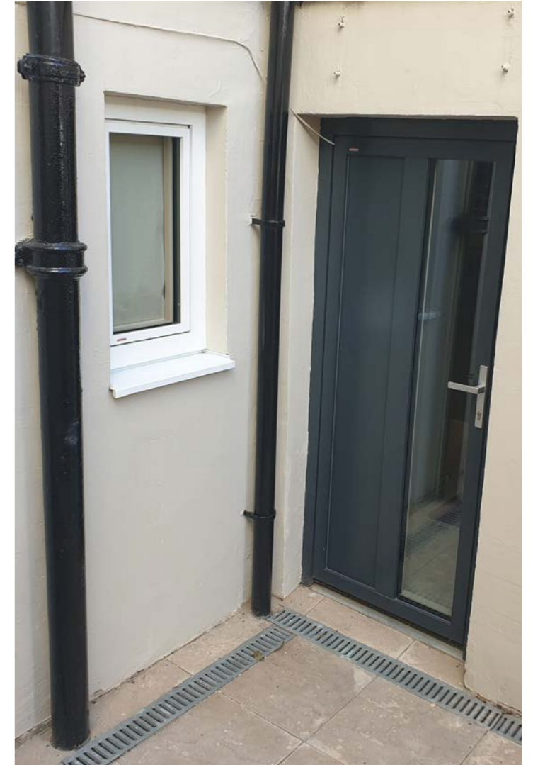
08 | View of side entrance at lower ground floor.
