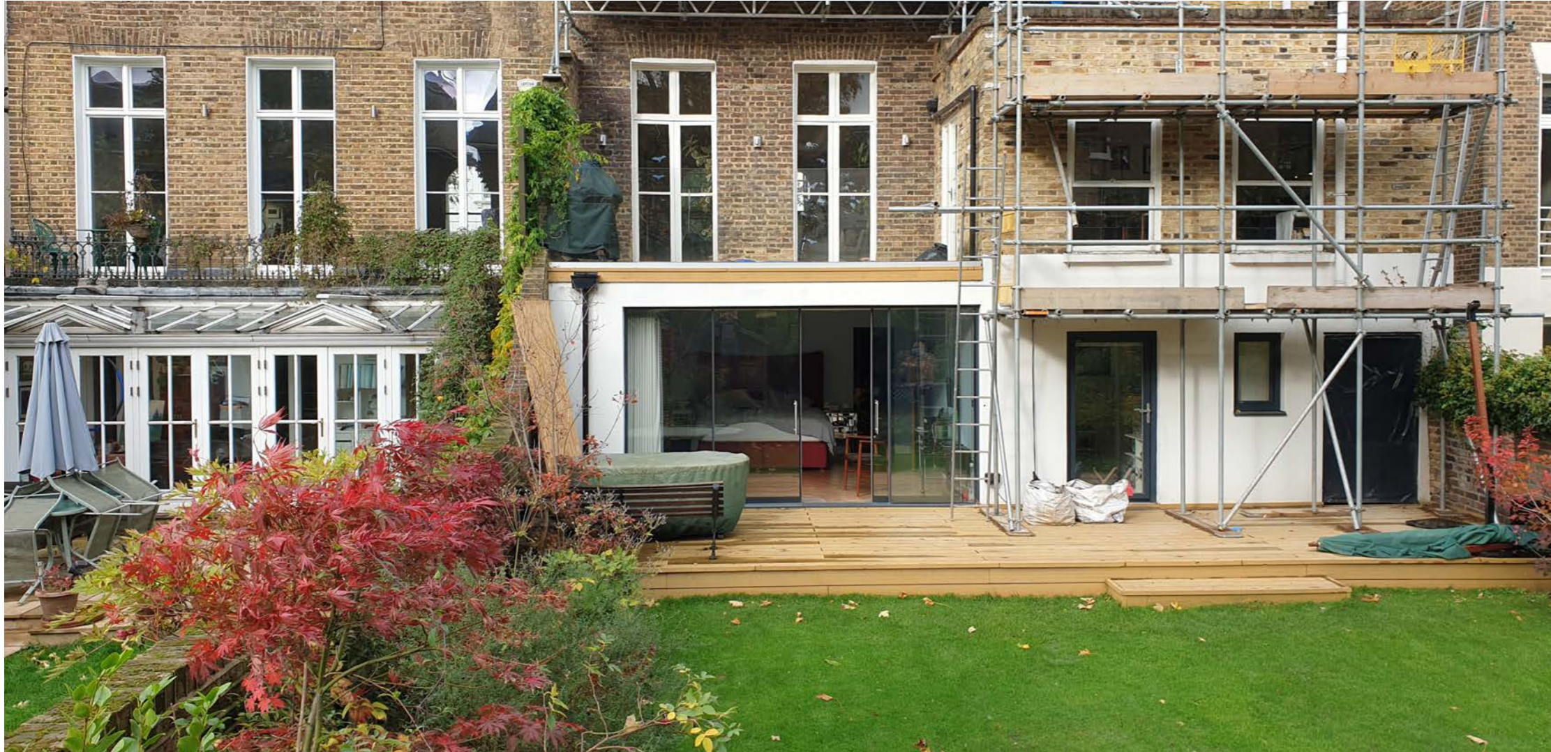
07 | No. 29 rear garden looking at the rear elevation in context of No.31 (L) and No.27(R). To the rear elevation of No.29, it is finished with white render at lower ground level. Powder coated aluminium slimline sliding doors to the south facing bedroom. The property presents some contemporary elements as existing. Photo taken during external decorative works early 2021.
