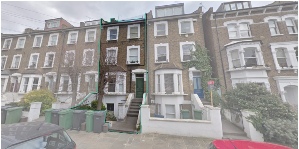
Figure 1. The Application Site
