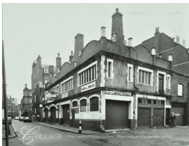
Figure 5. A photograph from 1978 looking south east at the corner of John's Mews and Northington Street. The Site is seen here as a closed and for sale Goodliffe Garages Limited. A number of external alterations had been
