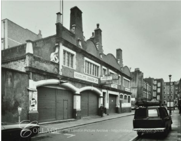
Figure 6. A photograph from 1978 looking south west along Northington Street. The image shows the building prior to further alterations in forming maisonettes at ground and basement levels, with lightwells created within the archways seen here to the left.
